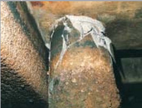
Clockwise from top left: Ground anchoring to stabilise quay, UK; Installing limpet dam to inspect and repair steel sheet piles below water level; Modification and repair of quay capping beam, Middle East; Replacement pile head ready for jacking into place; Accidental structural damage to concrete pile head, Malaysia.
