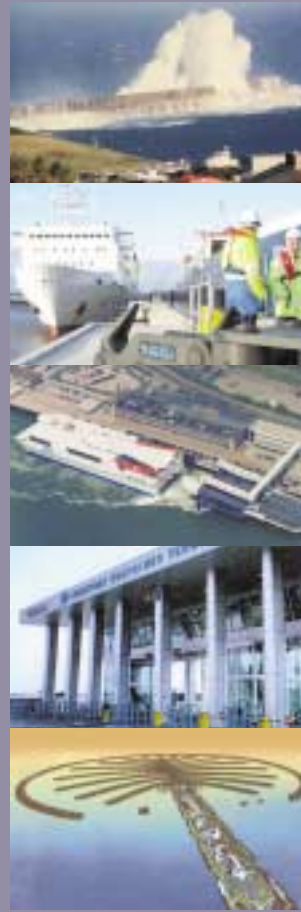
From top: Alderney Breakwater; Humber Sea terminal; HSS berth, Hoek van Holland, the Netherlands; West Port Container Terminal, Malaysia; Palm Island Development, Nigeria; Main image: Port of Dublin, Ireland.
